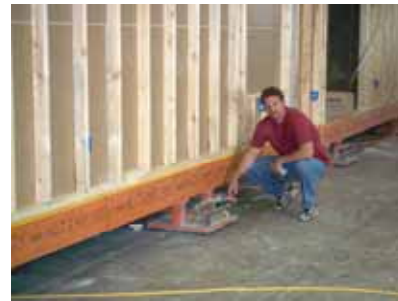
AeroGo Load Beams positioned under home frame.
